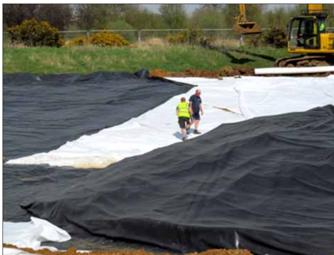
New lining being installed 24th April 2013
