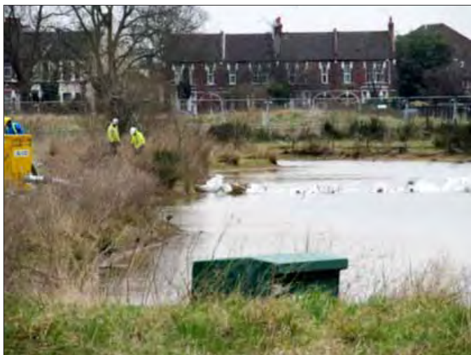
The dam, or bund, going across the narrowest part of the pond, 3rd April 2013
